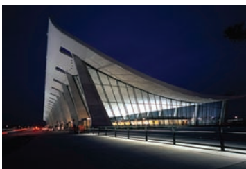
Roof of Washington Dulles Airport (hyperbola and parabola) Andrew Holt/Photographer's Choice/Getty Images
